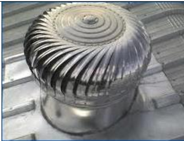
Figure 5.27. Powerless roof ventilator, Airier Natura Pvt. Ltd., Bangalore,
